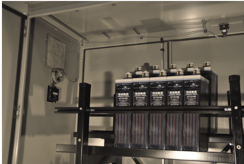
Batteries used in cellular base stations are usually placed in cabinets to protect the equipment.
